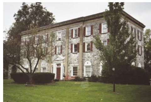
A $1.3 million renovation of Kappa Chapter has begun! The project is expected to be completed in August 2008.
